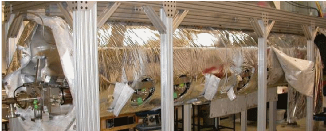
Figure 4.5.14: Photograph of the completed ERL injector 100 K shield being wrapped with MLI.
