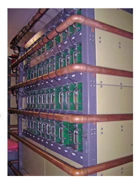
one for the klystron window and one for a window in the ring, a RF amplifier, and a PLC to keep track of everything, including interlocks and monitoring of directional couplers in the system.
