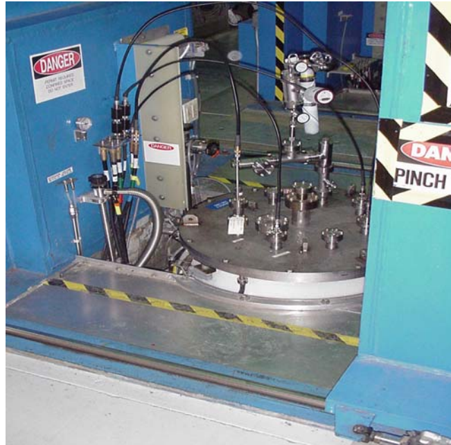
Top of a Vertical Test Dewar
