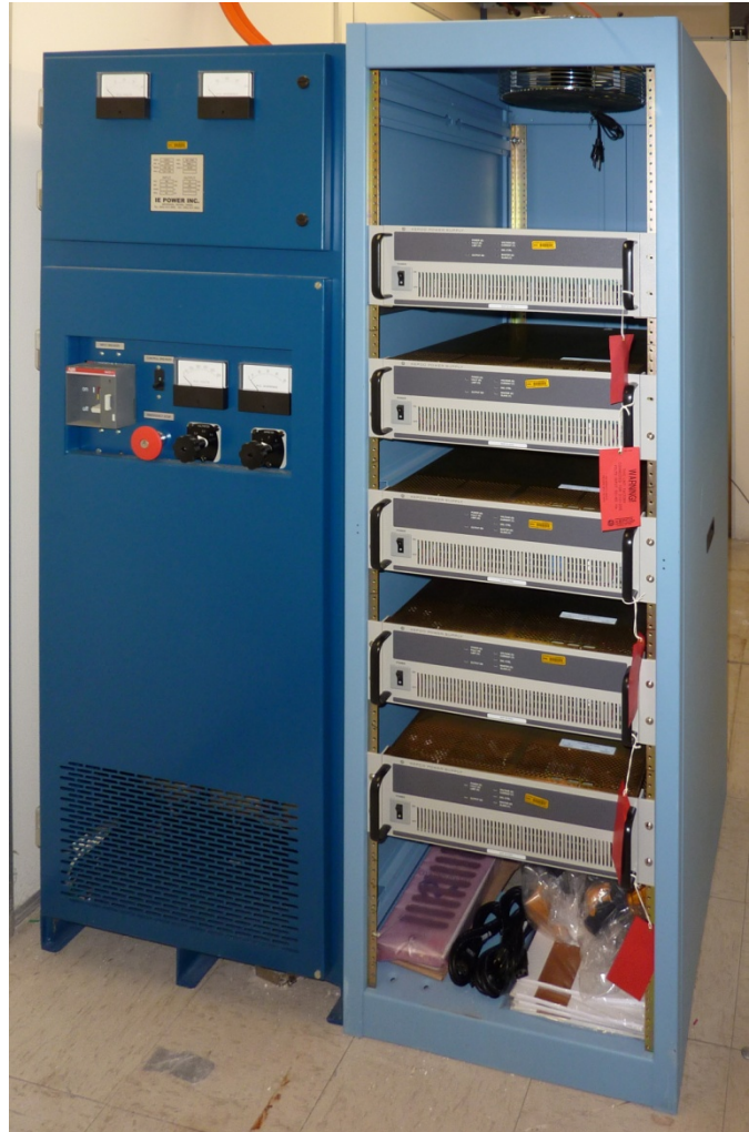
Figure 1. IE Power & Kepco Supplies
