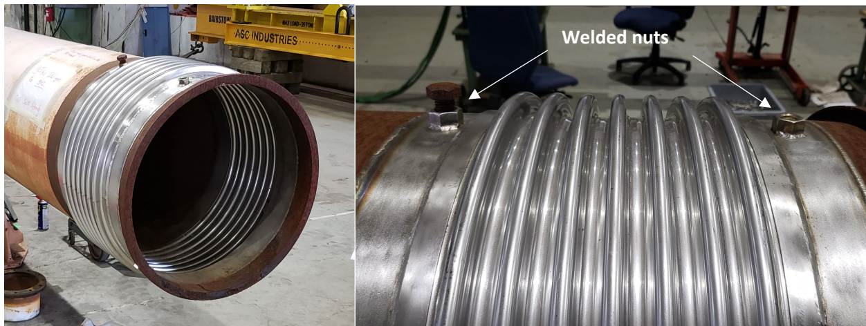
Figure 1 Bellow nut restraint installation
