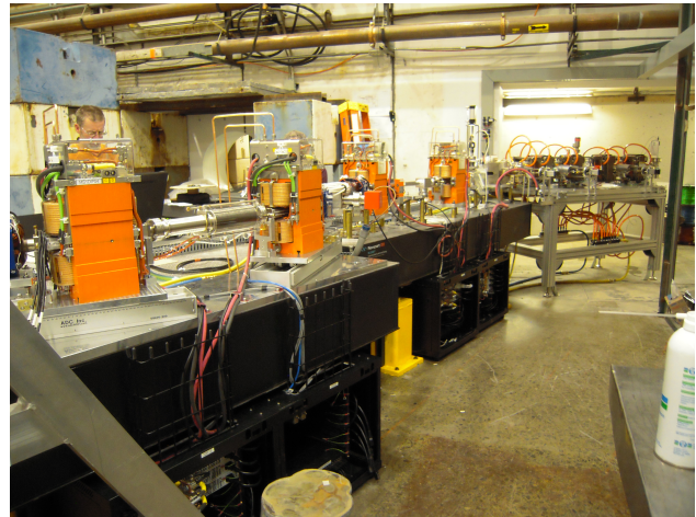
Figure 4: View from upstream of the splitter S1 line and the Splitter and FFAG cell magnets for the Fractional Arc Test.
