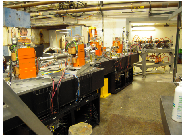
Figure 4: View from upstream of the splitter S1 line and the Splitter and FFAG cell magnets for the Fractional Arc Test.
